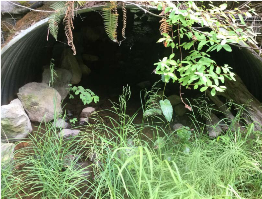
Outlet - nicely vegetated and stable
